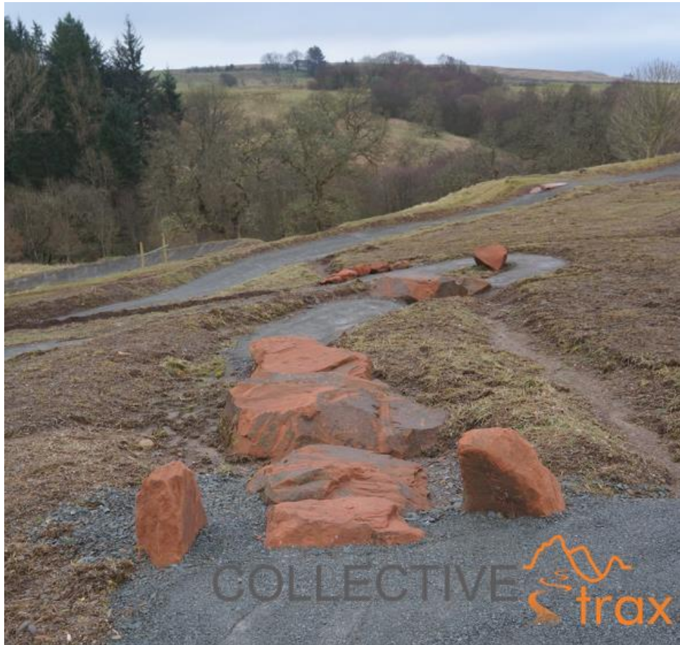
Image 16 - Technical Trail with Qualifier Feature. A Qualifier should be as technically difficult as anything else on the trail section, enabling riders to gauge the level of skill required prior to committing to the section.
