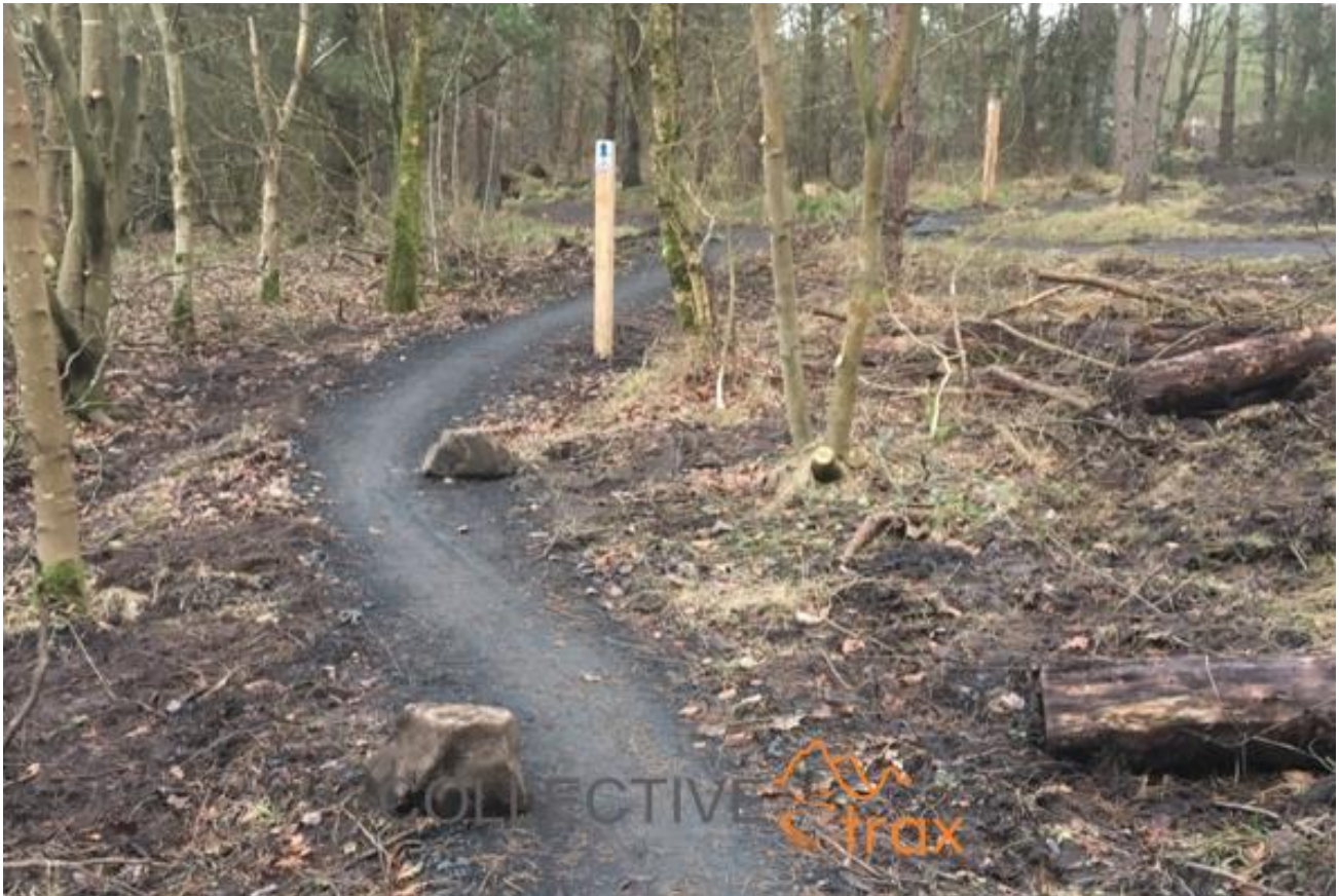
Image 12 - Path crossing example, utilising signage and a boulder chicane rather than pinch point.
