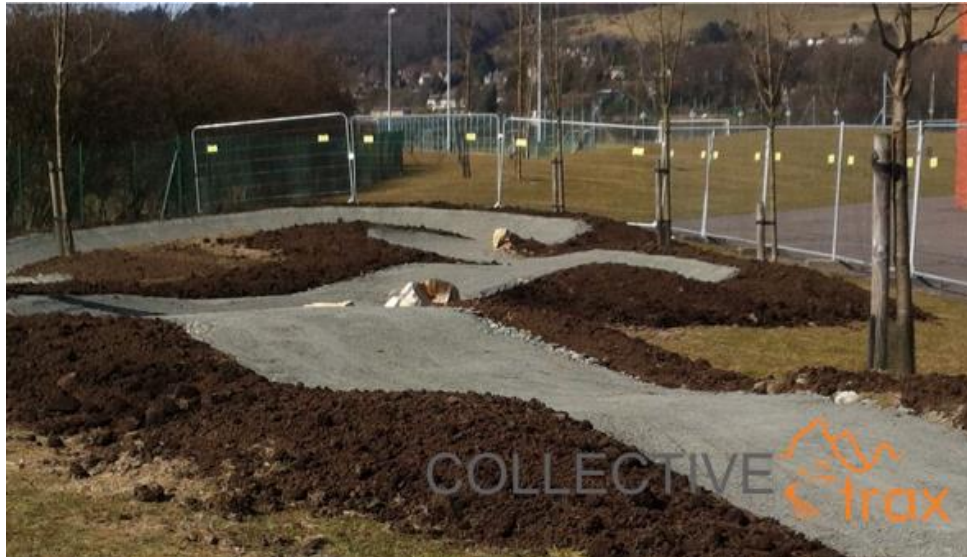
Image 17 – A newly built trail example. Soil dug out during construction is re-used to form bankings which support the trail and features.
